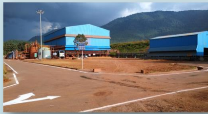
Red mud Filtration unit
