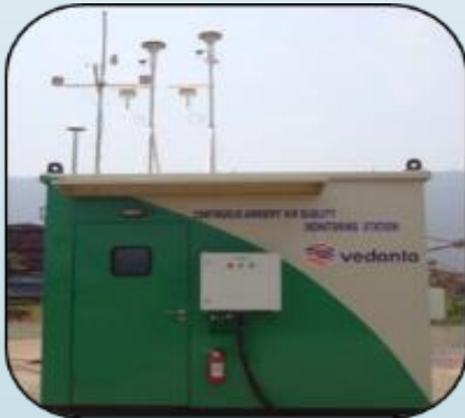
Continuous Ambient Air Quality Monitoring Station (CAAQMS)
