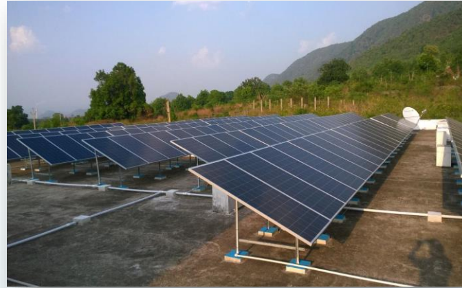
Solar Power station 180 Kw peak in refinery and and 200 Kw peak in township
