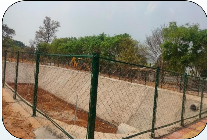
Rainwater Recharging Structure in Township to recharge more than 1 lakh m3 of water
